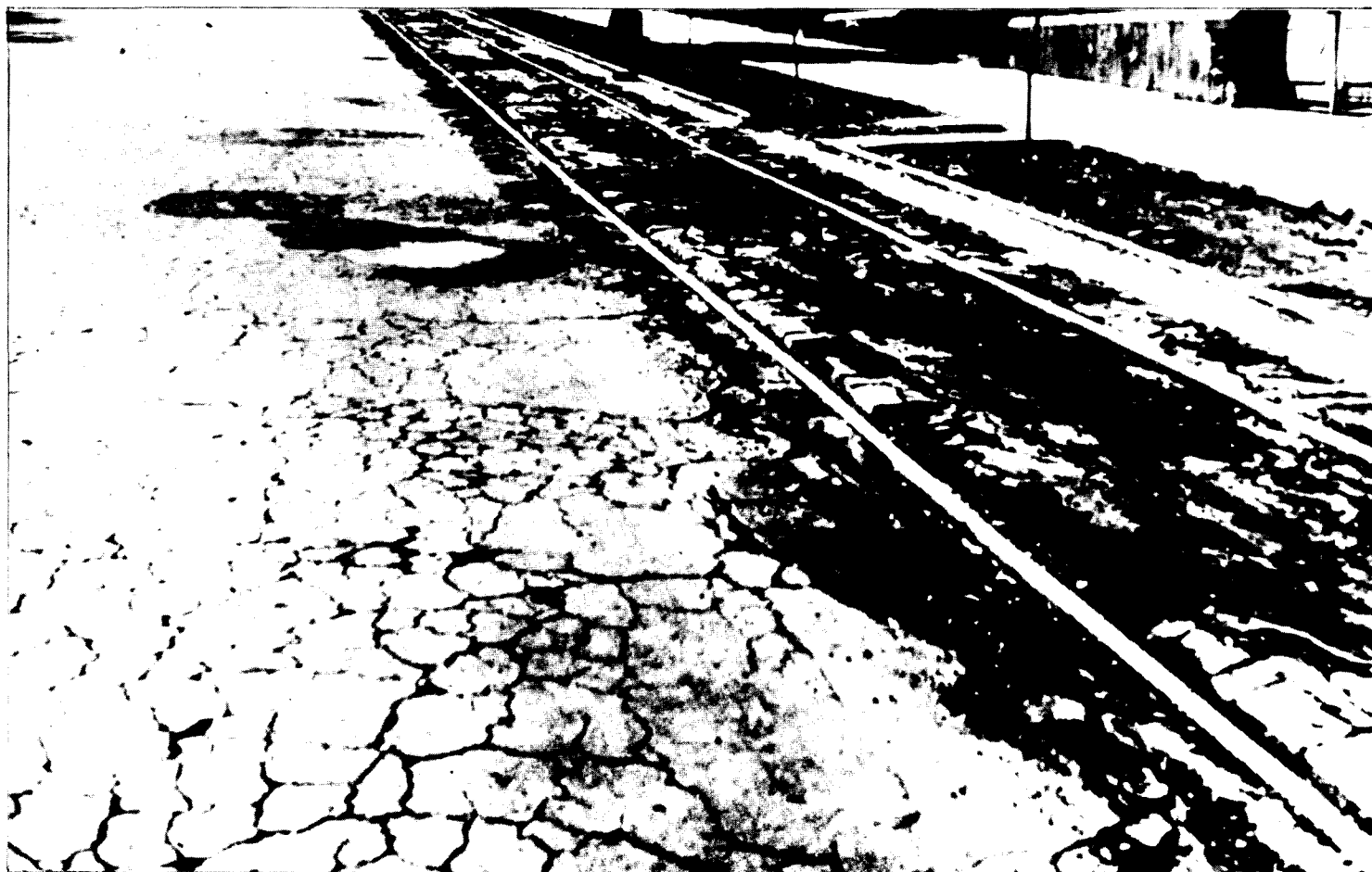
FIGURE 1: APPEARANCE OF AN ASPHALT PAVEMENT THAT WAS MADE WITH A HARD VOLCANIC PUMICE AGGREGATE
