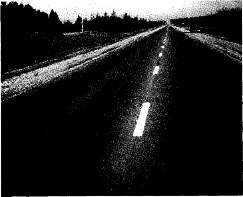
Figure 24: Pavement with 150/200 Penetration Asphalt. West of Orangeville. Four Years Old.
