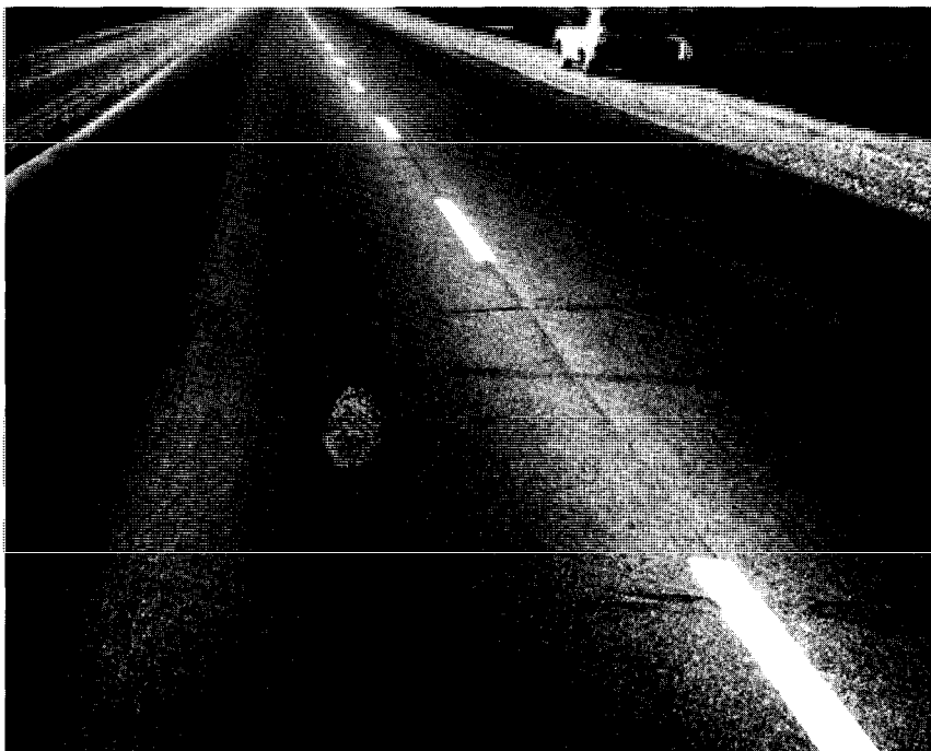
Figure 25: 85/100 Penetration in Pavement in Right Lane. 150/200 Penetration in Left Lane. West of Orangeville. Four Years Old. (Note: Blemish is in the Film Not in the Pavement).
