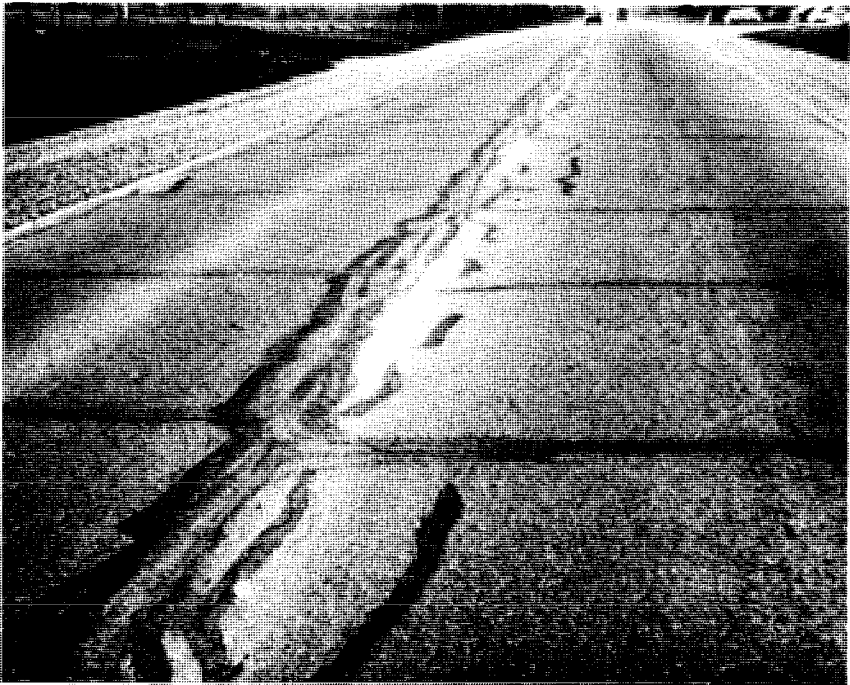
Figure 23: Pavement with 85/100 Penetration Asphalt. West of Orangeville. Four Years Old.
