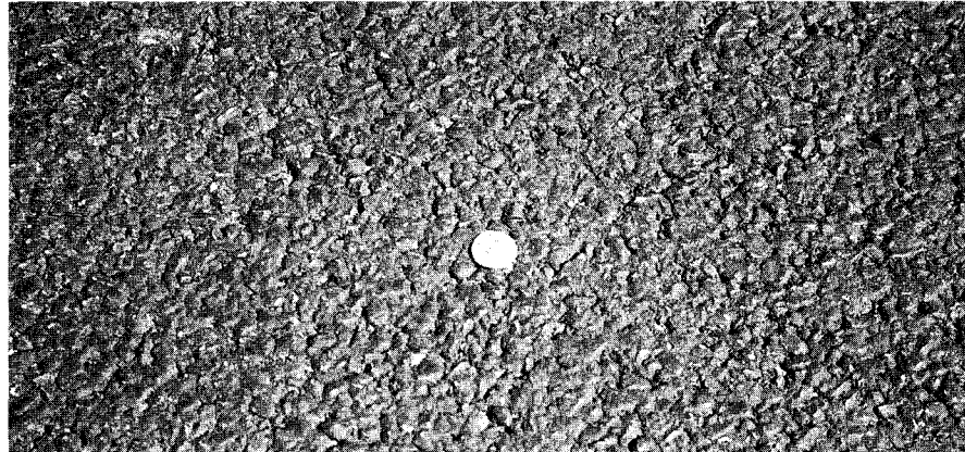
PHOTOGRAPH 8. CLOSE-UP OF STONE MASTIC ASPHALT (SMA 3) SURFACE TEXTURE AFTER FIVE WEEKS.
