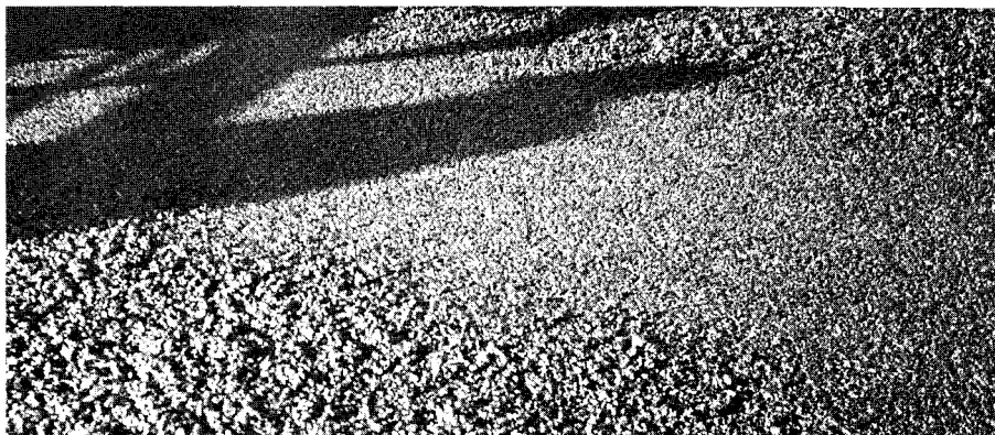
PHOTOGRAPH 3. GENERAL APPEARANCE OF SMA 1 MIX AFTER PLACEMENT AND IN AREA WITH ONE PASS OF STEEL-WHEEL ROLLER.
