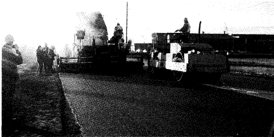
PHOTOGRAPH 2. PLACING OF STONE MASTIC ASPHALT (SMA 1) IN DECEMBER 1990.
