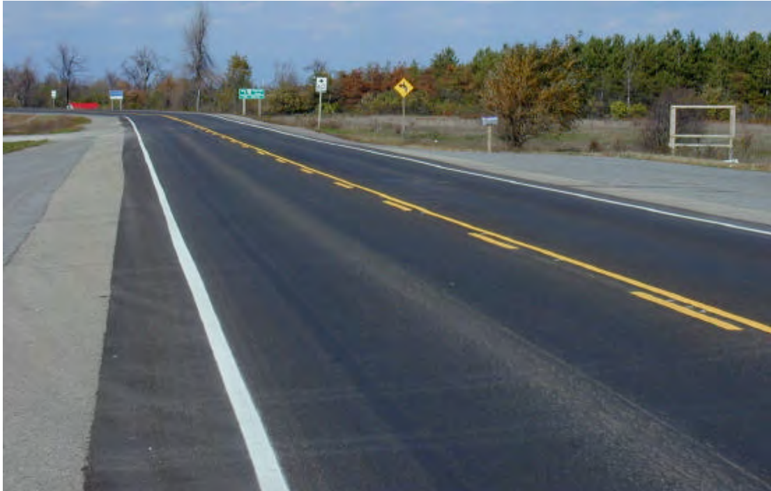
Figure 7. Micro-Surfacing after a few months of service
