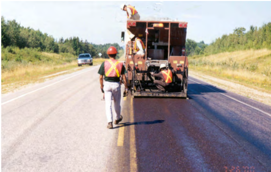
Figure 6. Rut Filling Operation
