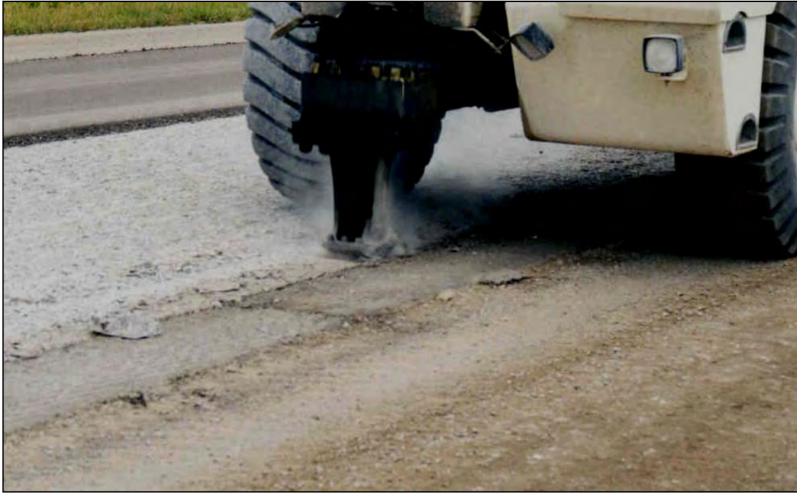
Photograph 6: Resonance breaker shoe
