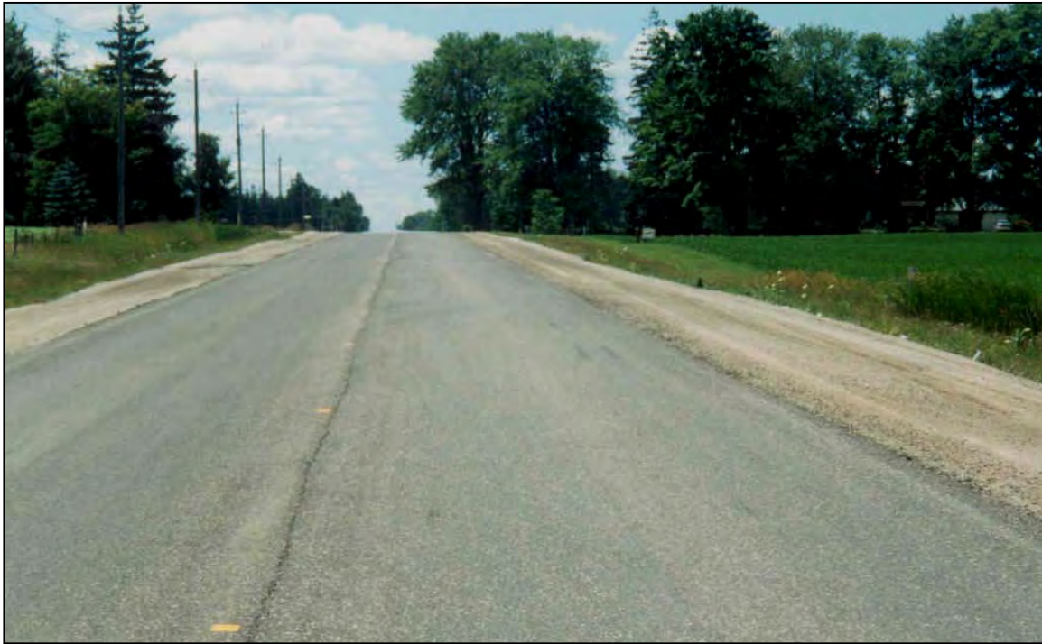
Photograph 9: Cured stockpiled recycled cold mix
