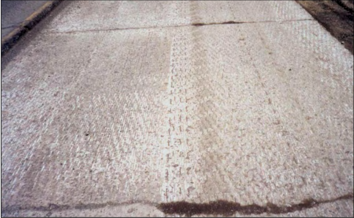
Photograph 4: Milled surface of concrete slab before rubblization
