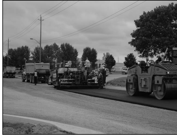
Figure 2b: Placement of HL8 RAP Mix
