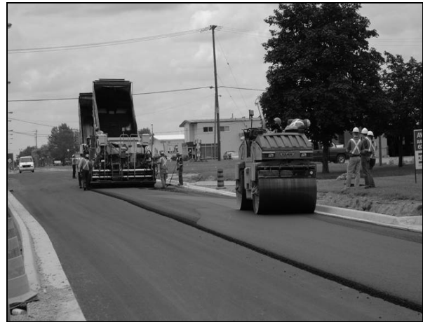
Figure 4d: Placement of Second Lift
