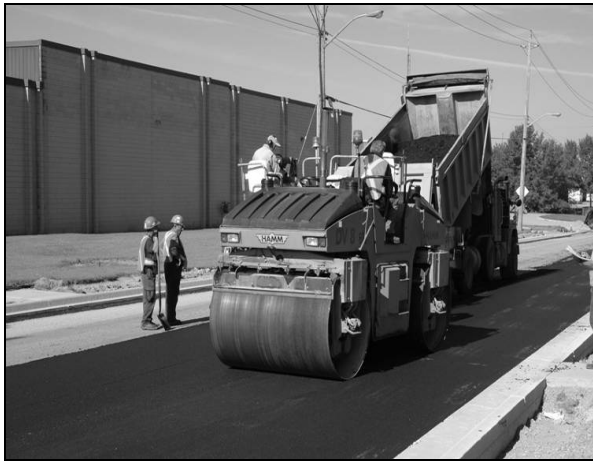
Figure 4a: Placement of Bottom Lift
