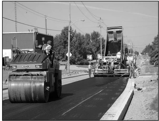
Figure 4b: Rolling First Lift of HL8 RAP Base
