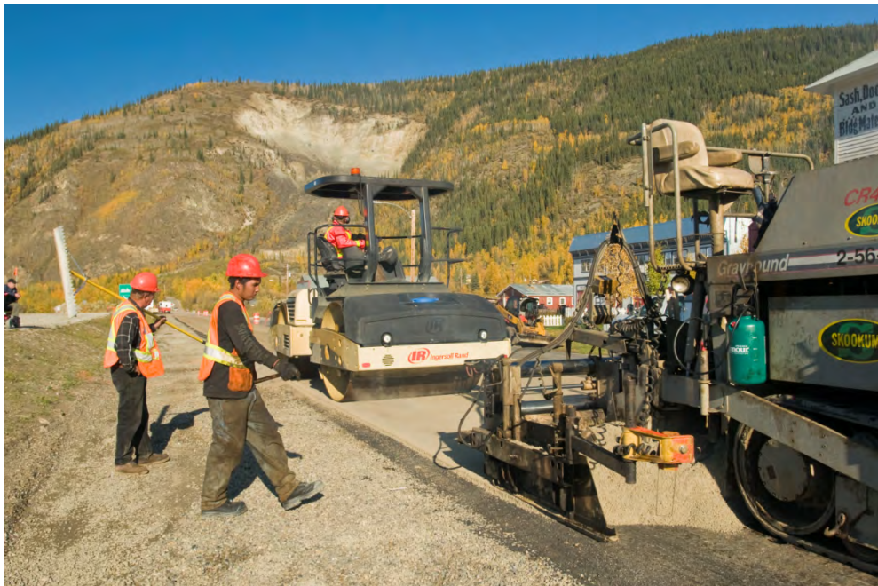
Figure 2. Paving Operation, Dawson City, Yukon, September 2009
