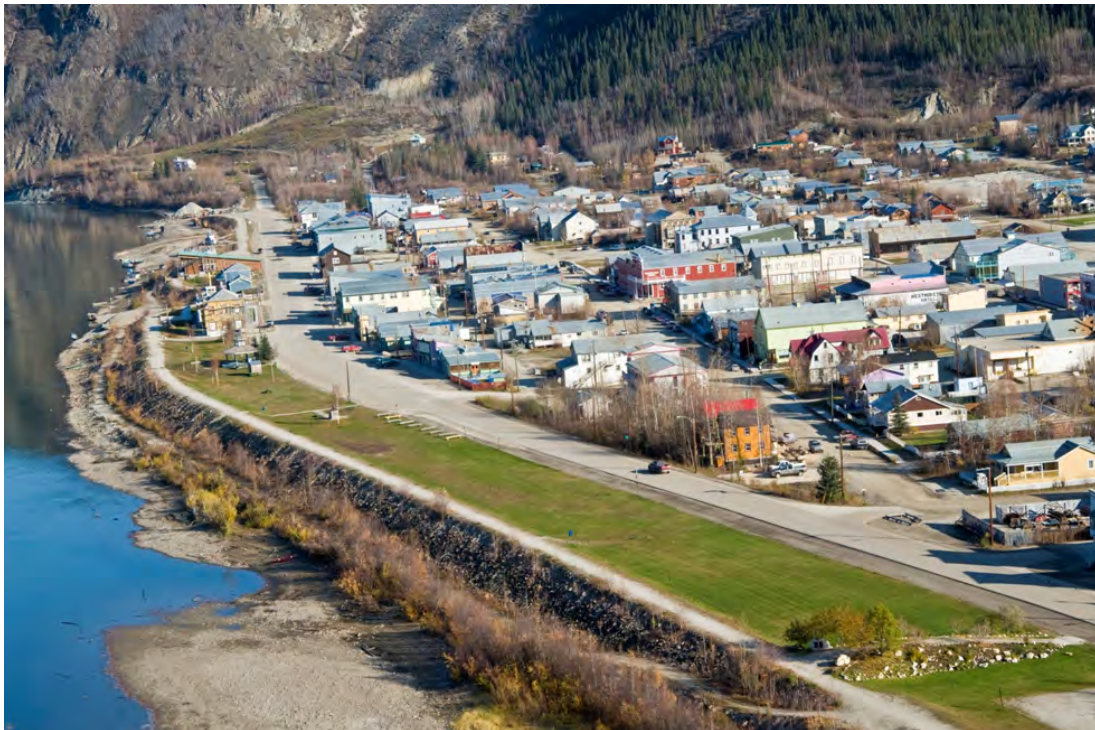
Figure 4. Aerial View of Front Street, Dawson City, Yukon, September 2009
