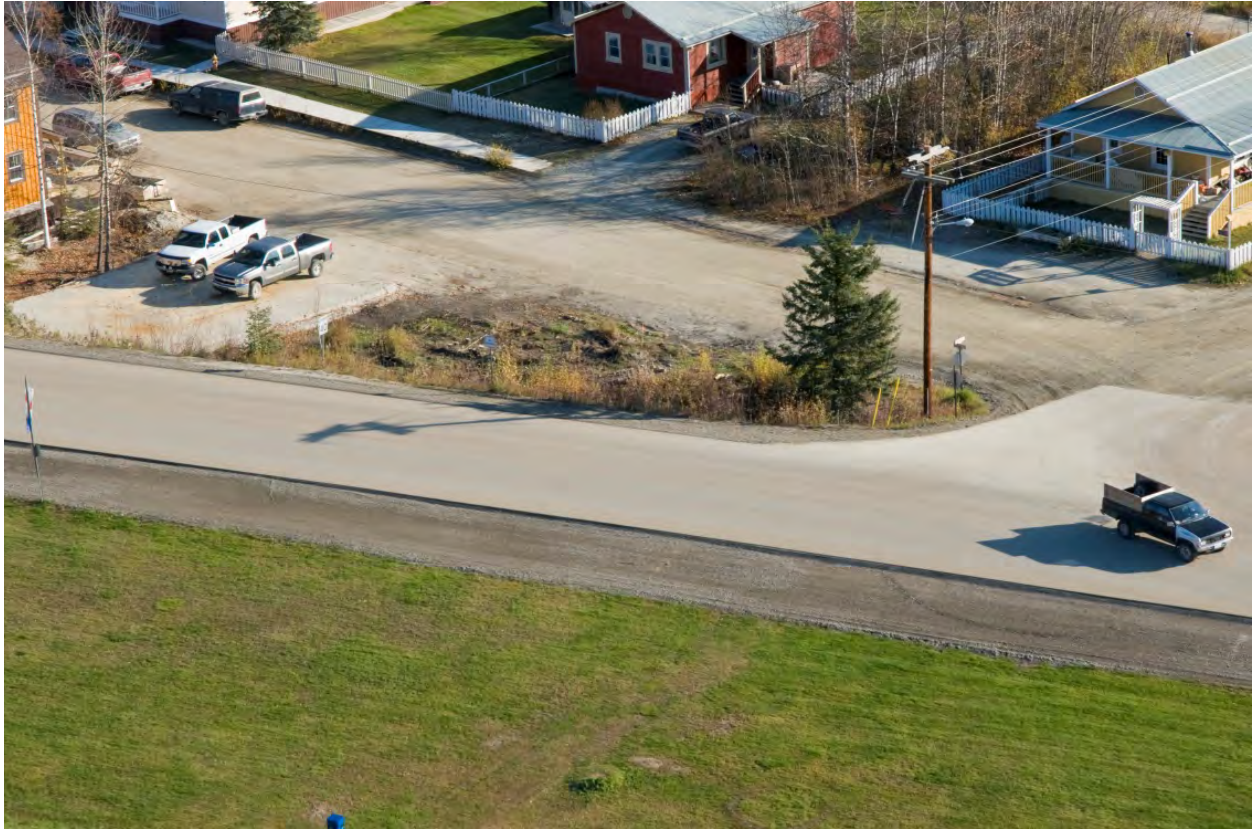
Figure 6. Light-coloured Pavement in Comparison to Surrounding Gravel Surfaces
