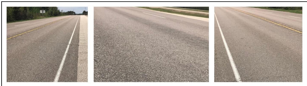
Figure 7. Highway Section Completed Using Job Mix D III in Eastern Manitoba
