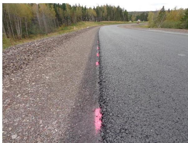
Pic 11: Primed area not shoving laterally; Paint line guide is gone. Paint line guide line is still exposed
