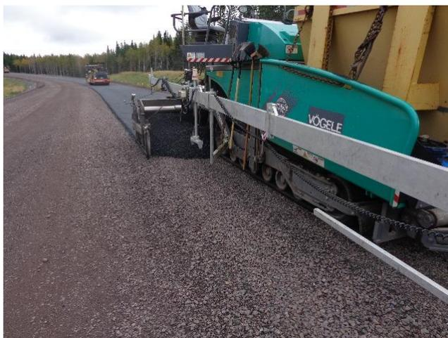
Pic 12: Paving over a loose unprimed granular surface
